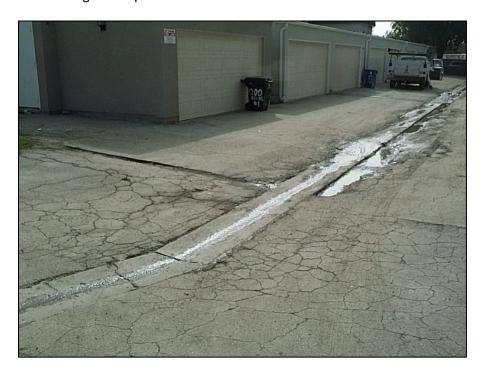
The driveway pictured above belongs to an Association that thought they were saving money by not seal-coating their asphalt. That decision led to complete premature failure of their entire driveway system. In addition to being unsightly, the ensuing "remove & replace" project will cost about 10 times as much as that less expensive seal coat project they failed to perform a few years ago.
