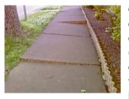
Concrete can be expected to last an extended period of time. But over time, most concrete walkway installations will require repairs or replacements. Concrete is by nature strong in compression (when a load is placed on it), but it is brittle (its edges are prone to cracking and chipping, and it will crack when exposed to repeated freeze/thaw cycles) and it cracks easily when subjected to bending loads. So when it is flat in the ground it will last a long time. But
