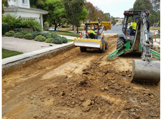
THE RESULT OF POOR MAINTENANCE
